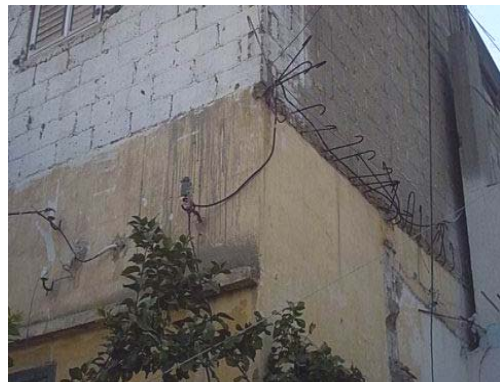
Fig. 4.9: Local Spalling of Concrete Cover.
