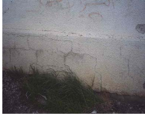
Fig. 4.13: Vertical and Inclined Cracks in Bearing Walls under Ground Beams.
