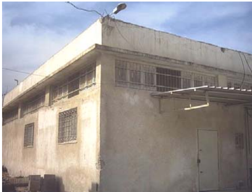
(a) An old building in Gaza. (Shifa Hospital)
