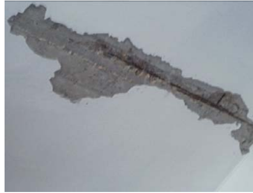
Fig. 4.9: Local Spalling of Concrete Cover.
