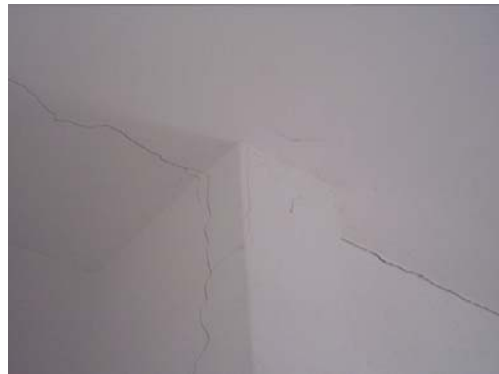
Fig. 4.13: Vertical and Inclined Cracks in Bearing Walls under Ground Beams.
