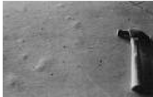
Blistering (www.structuraldesigns.com.au)
