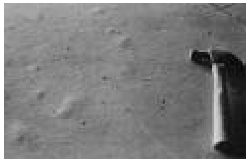
Blistering (www.structuraldesigns.com.au)
